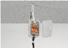
Pendant light connection in a suspended ceiling
